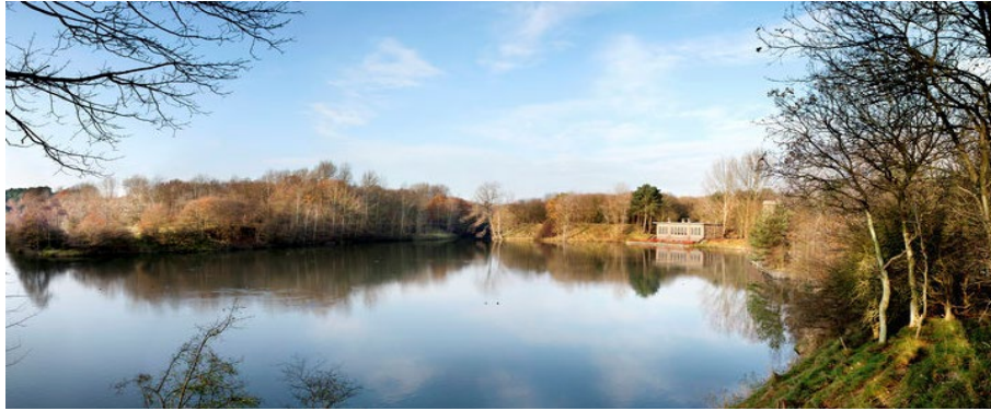
Figuur 1C: Pompstation Oranjekom
